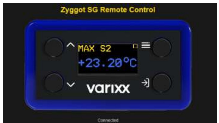
REMOTE CONTROL AND DATA READING BY ETHERNET
