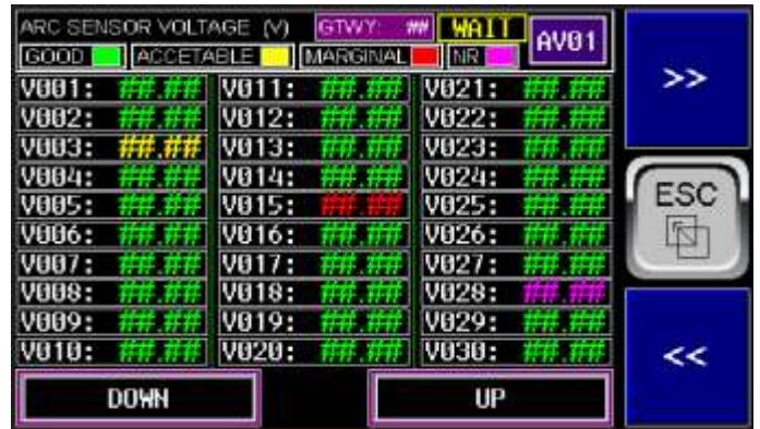
ARC SENSORS VOLTAGE LEVEL AV01 a AV04:
